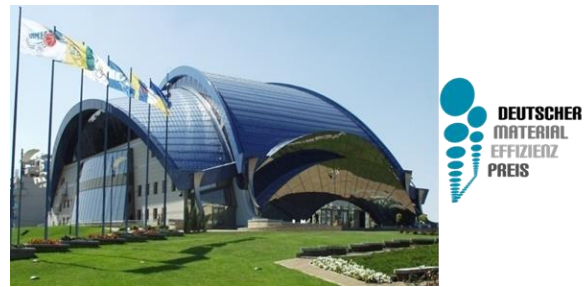
Figure 16 : Vault-structured roof in Odessa (Böhme Haustechnik)
