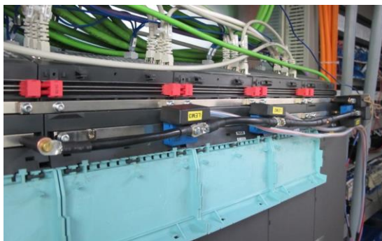
Figure 3: Mounted Hall-effect current sensors for measurement on the DC link to drive inverters.
